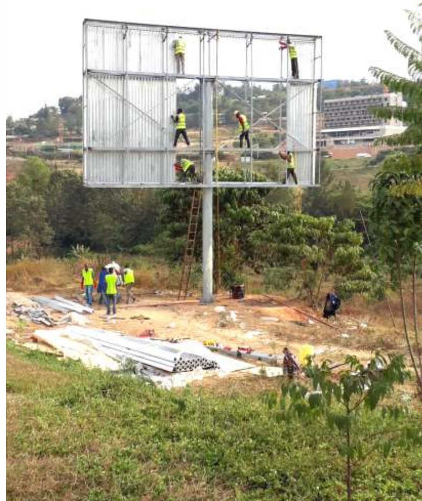
ROTAPANEL TRIVISION INSTALLATION IN KIGALI, RWANDA.
