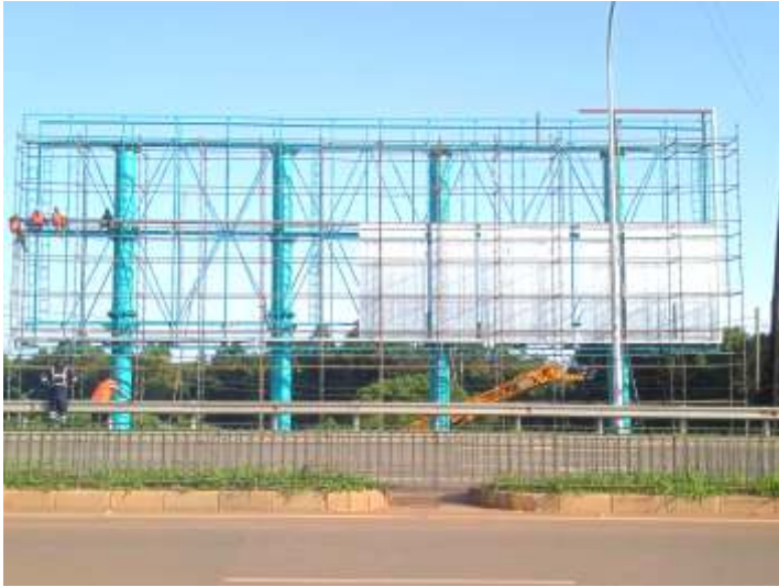
ROTAPANEL TRIVISION INSTALLATION IN KAMPALA, UGANDA.
