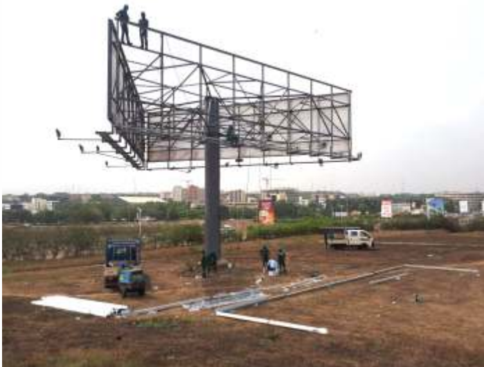
ROTAPANEL TRIVISION INSTALLATION IN ACCRA, GHANA.
